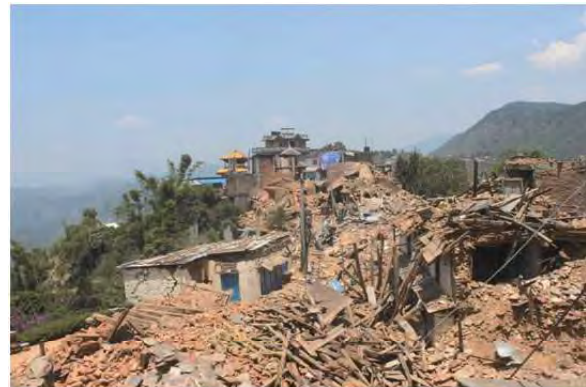
Photo. 1 Old Chautara town on ridge and damaged houses
