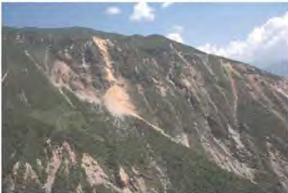
Photo. 3 Shallow failures in Sindhupalchowk district
